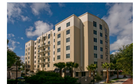
Orlando Lutheran Tower
